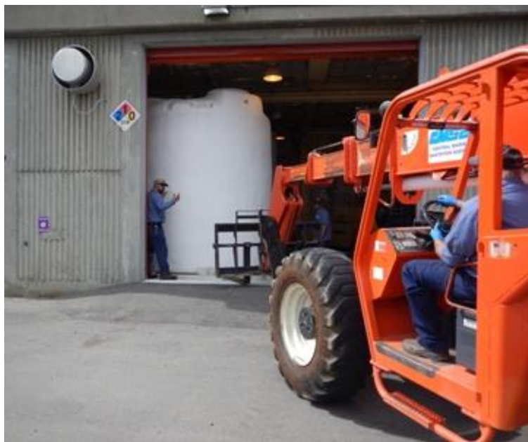
Moving the new Hypochlorite Tank into the Chemical Storage Building.
