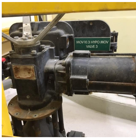
Originally Installed Valve.
