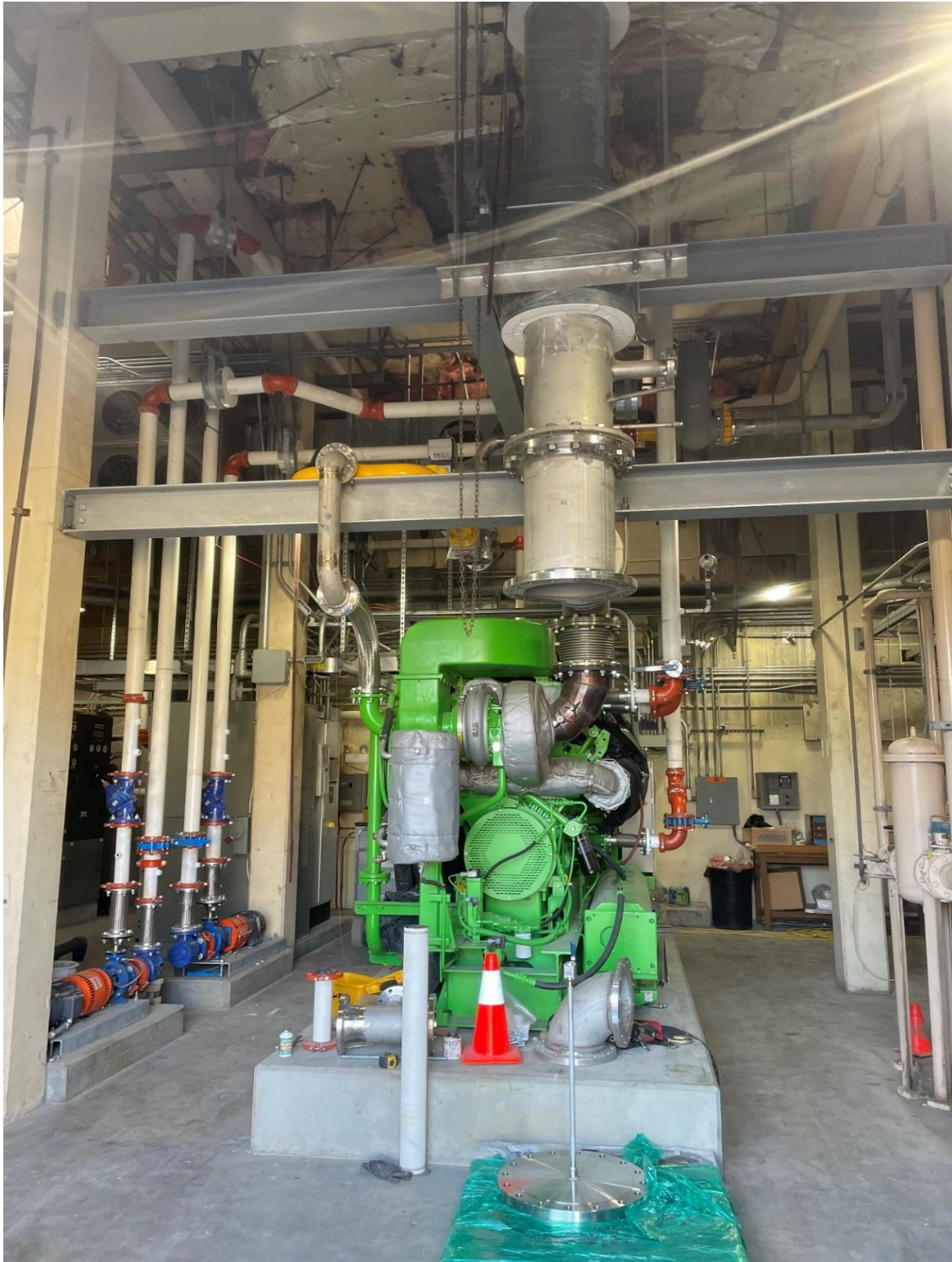
New cogeneration engine in final installation phase.
