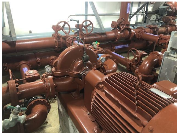
Originally installed Recycled Water Pump.
