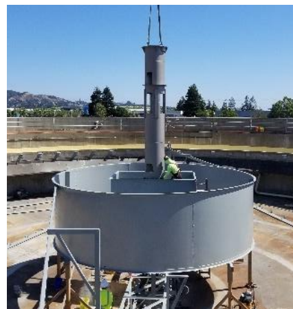
Installing new center column/RAS pipe.
