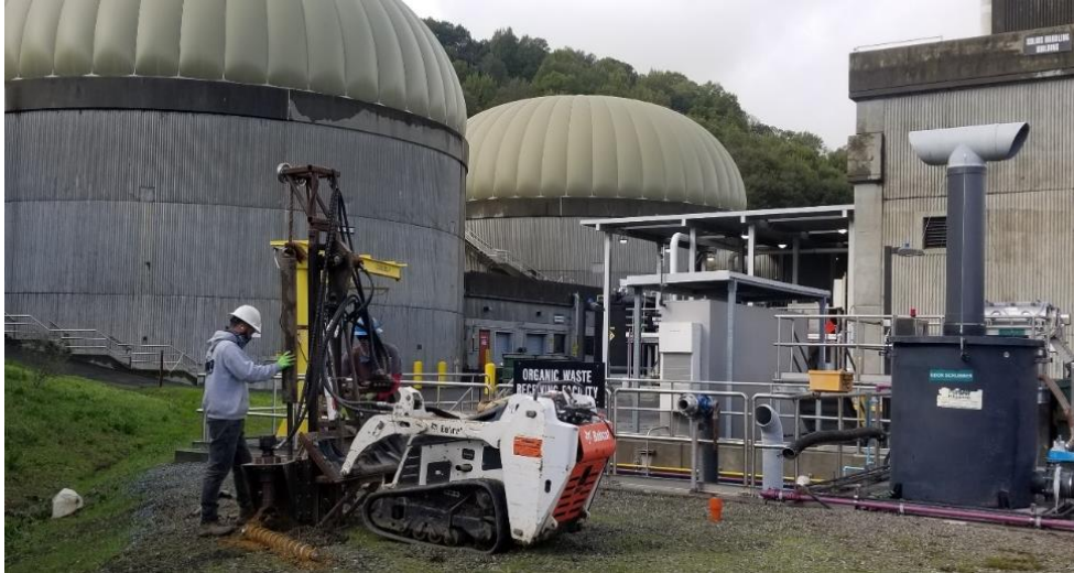
Geotechnical boring for new above-grade storage tank location.
