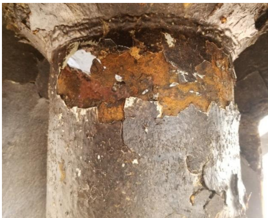
Old center column/RAS pipe.
