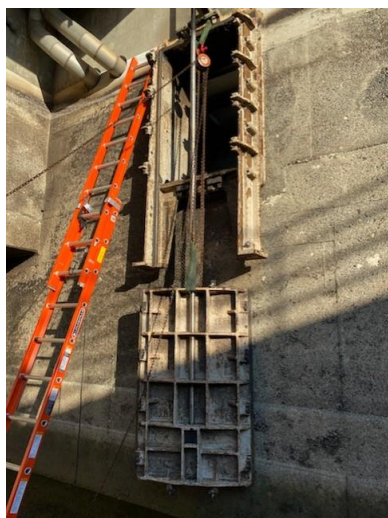
Originally installed Cast Iron Influent Gate
