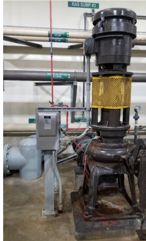
Existing RAS pump.
