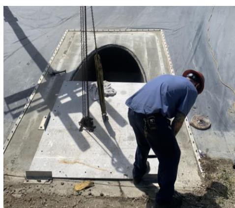
Technician blanking of pipe.
