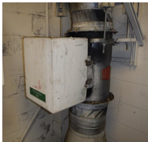
Existing Exhaust Fan.
