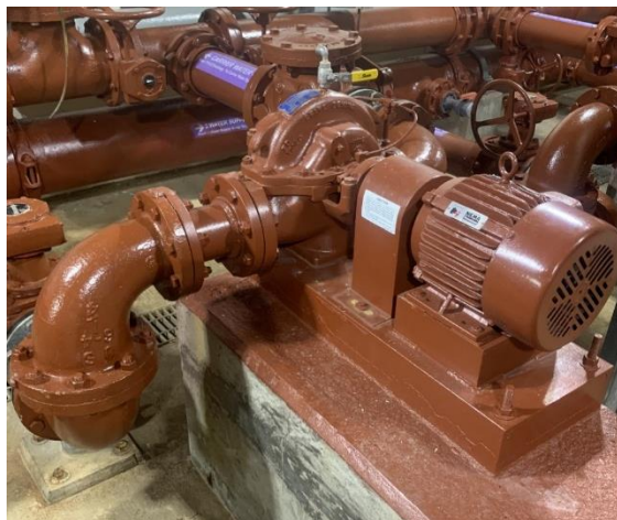
New Recycled Water Pump.
