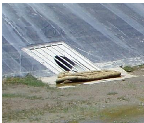
Originally installed pipe.
