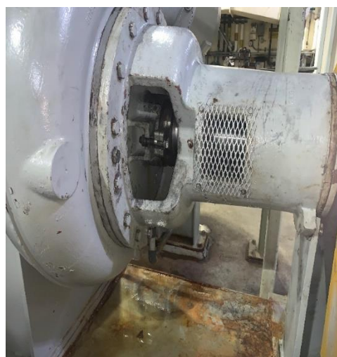
Reassembled and Refurbished Biotower Pump.
