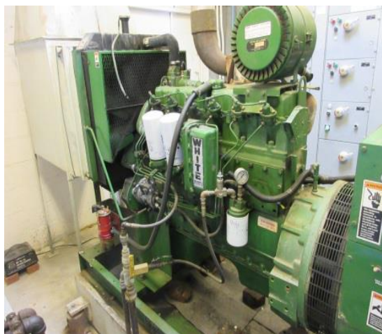
Existing Emergency Generator.
