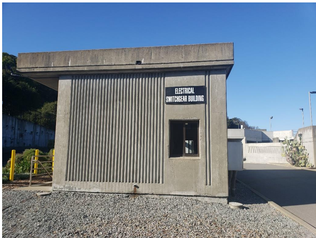
CMSA's Main Facility Switchgear Building.
