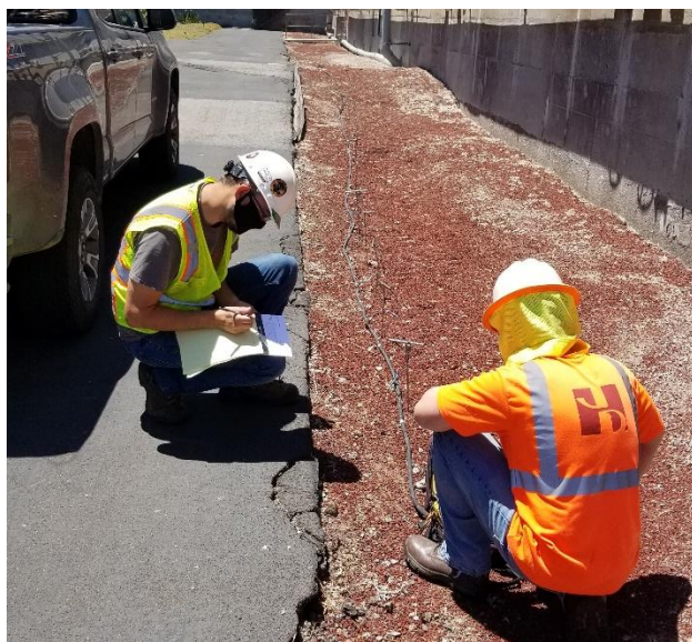
In-situ soil resistivity test.
