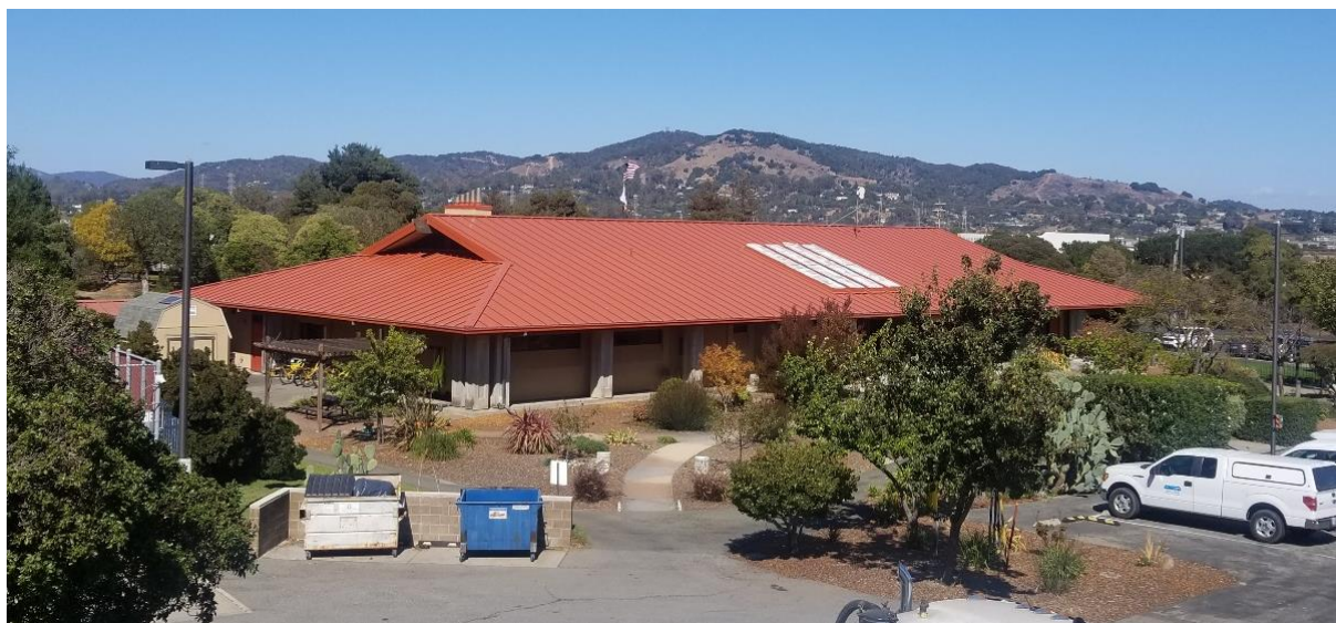
New metal panel roof and skylight framing.
