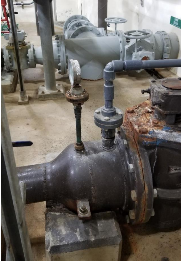
Corrosion on existing RAS piping.
